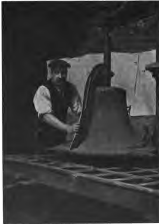
FIG. 199.—Striking up Core for Bell.
